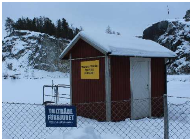
Fig. 17. Pumphouse and water protection zone sign.
