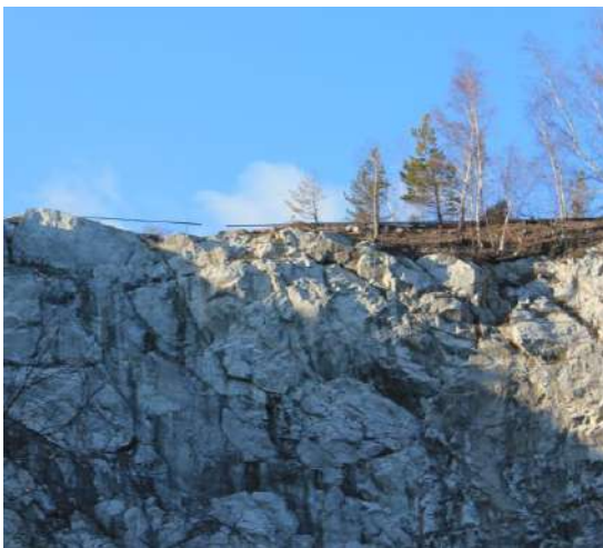
Fig. 12. The residues of old water system.
