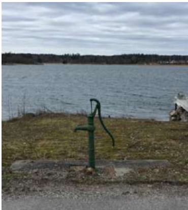
Fig. 23. Old manual water pump.
