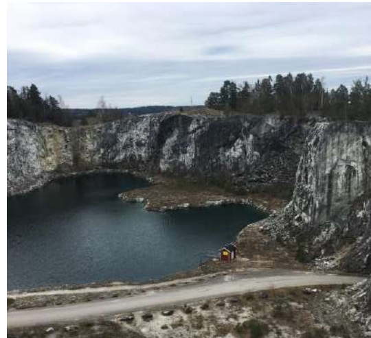
Fig. 13. Pumphouse for major water intake.
