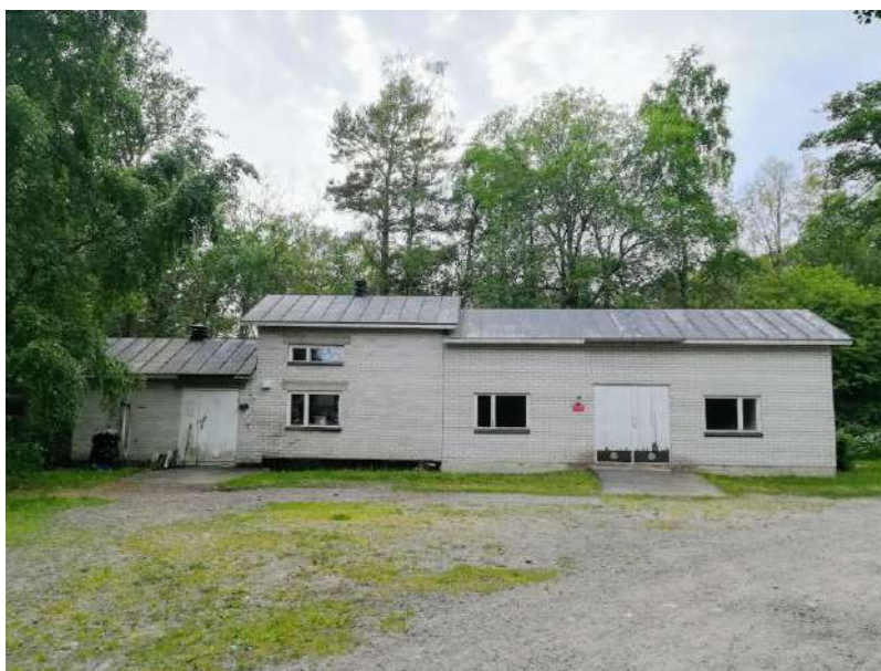
Figure 12. The water purification plant in Öro. (Picture: Lotta Eriksson 2019)
