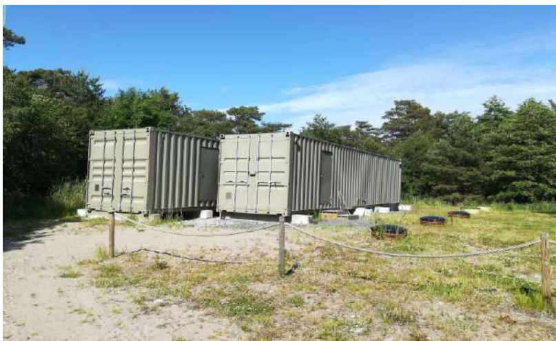
Figure 16. The wastewater treatment plant in Örö. (picture Lotta Eriksson 2019)
